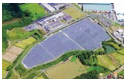
Noboribetsu, Japan 22MW Solar Power Station
