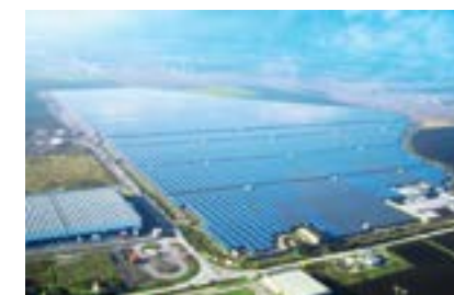
Rovigo 70MW Solar Power Station
