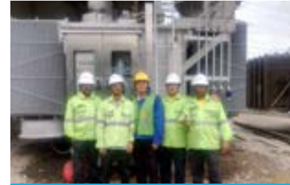
Rawang Lafarge Cement Plant, 132kV Transformer
