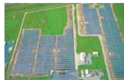
CA Depot Park, USA 3MW Solar Power Station
