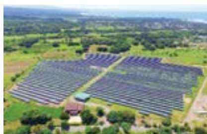
Bataan, Philippines 5MW Solar Farm Project
