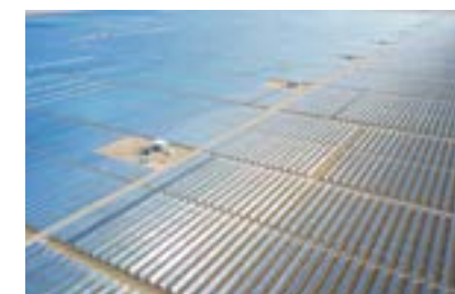
Sakaka, Saudi Arabia 405MW Solar Power Station
