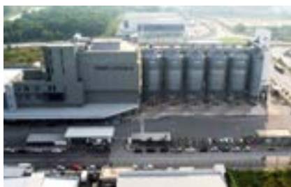
Penang Federal Oats Mills Factory
