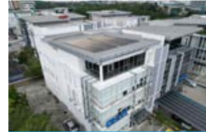
Selangor 37.4kWp Solar PV Industrial Project
