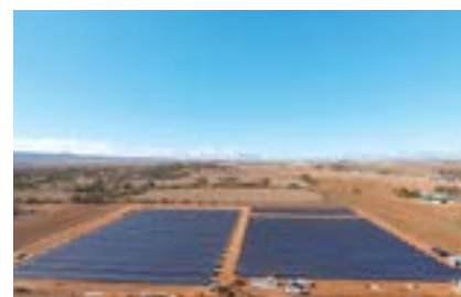
Bungama, Australia 1.88MW Solar Power Station
