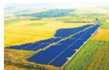
Ezmer 10MW Solar Power Station
