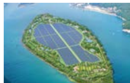
Korea Boongeo 9MW Solar Power Station
