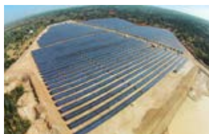
Thailand EPD 16MW Solar Power Station
