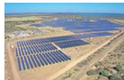
Limpopo, South Africa 64MW Solar Power Station
