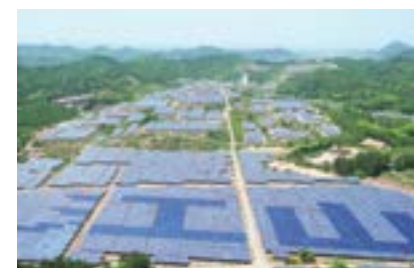
Jiangshan Agriculture Complimentary 200MW Solar Power Station
