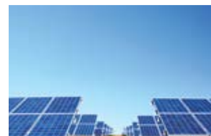
Kings Mountain, USA 8MW Solar Power Station
